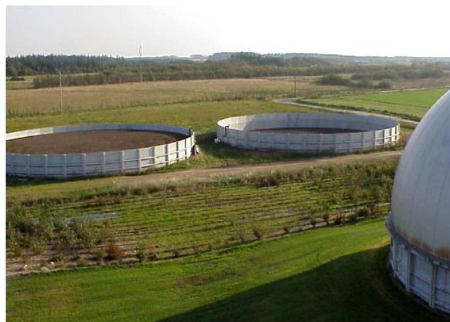
Figure 7.32 Storage tanks covered with natural floating layer (DANISH BIOGAS ASSOCIATION 2008)
