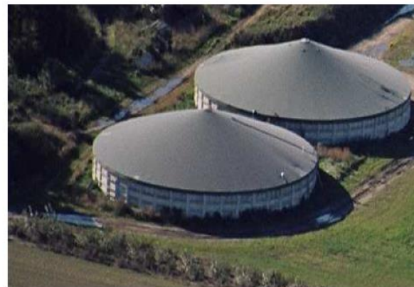
Figure 7.33 Membrane covered storage tanks (DANISH BIOGAS ASSOCIATION 2008)
