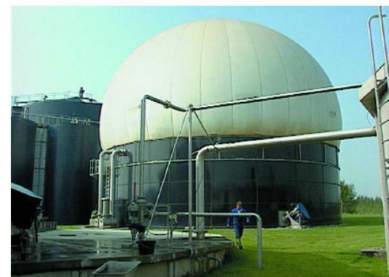
Figure 7.33 Membrane covered storage tanks (DANISH BIOGAS ASSOCIATION 2008)
