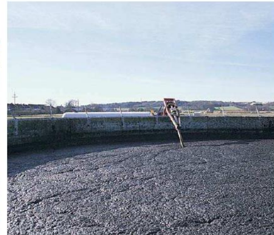
Figure 7.32 Storage tanks covered with natural floating layer (DANISH BIOGAS ASSOCIATION 2008)
